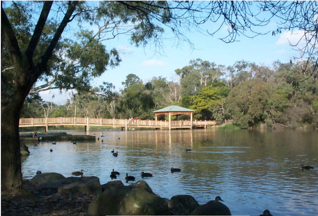
Restored lake bridge - 2000
