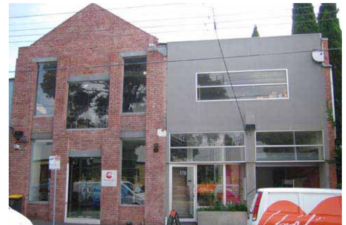
Sensitive Interface between New and Existing Buildings
