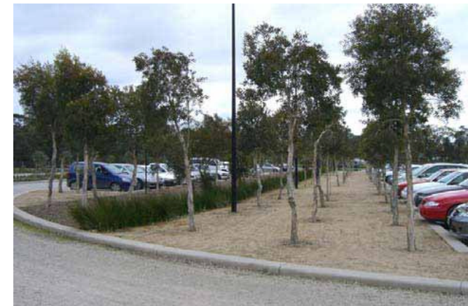
Example of water sensitive urban design in a car park
