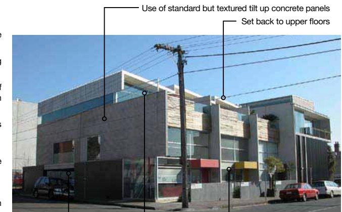
Use of standard but textured tilt up concrete panels Set back to upper floors Clear entrances Good, clear lower and upper floor glazing Underground car parking to side street
