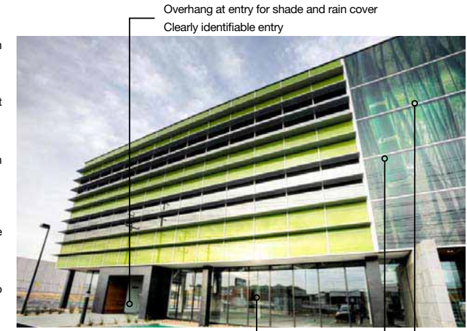
Overhang at entry for shade and rain cover Clearly identifiable entry Clear glazed lower windows High quality facade treatment with additional louvers to north aspect Transparency in upper floors so activity can be seen
