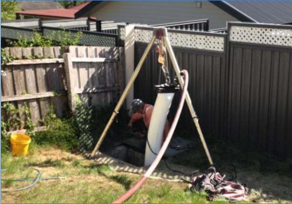
Figure 6 - Council contractor performing drainage relining works via a pit in an easement at the rear of a property
