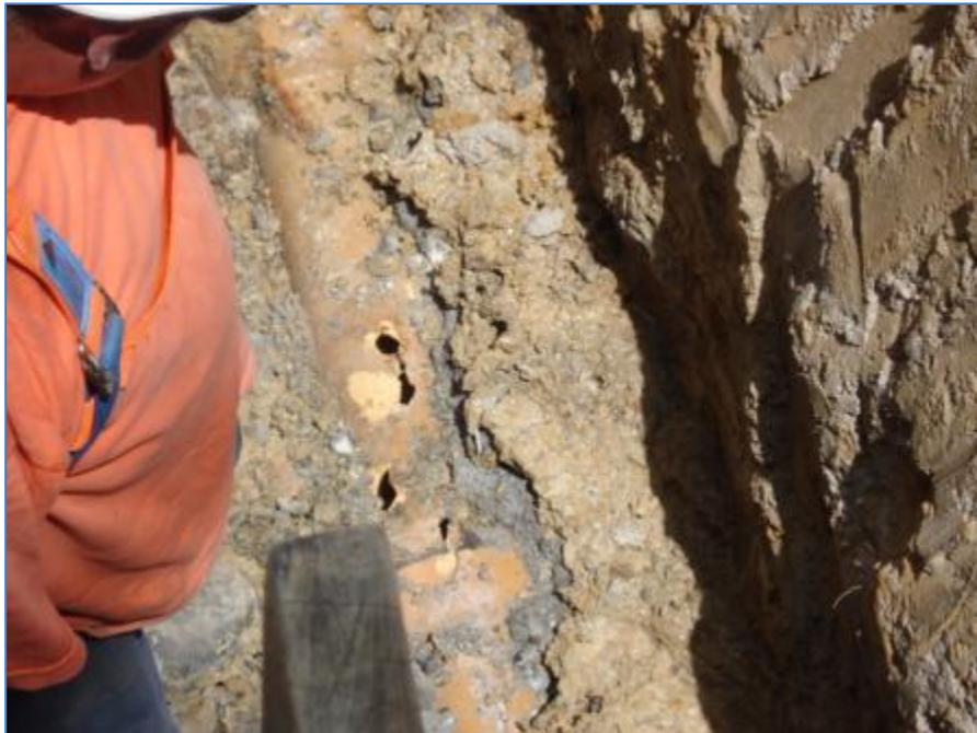
Figure 19 - a broken (old) terra cotta drain in an easement that needs replacing
