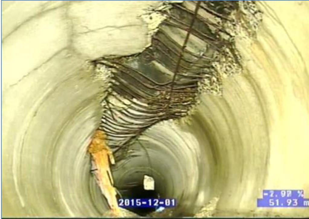
Figure 20 - an internal view of a drain that has failed and collapsed due to loading
