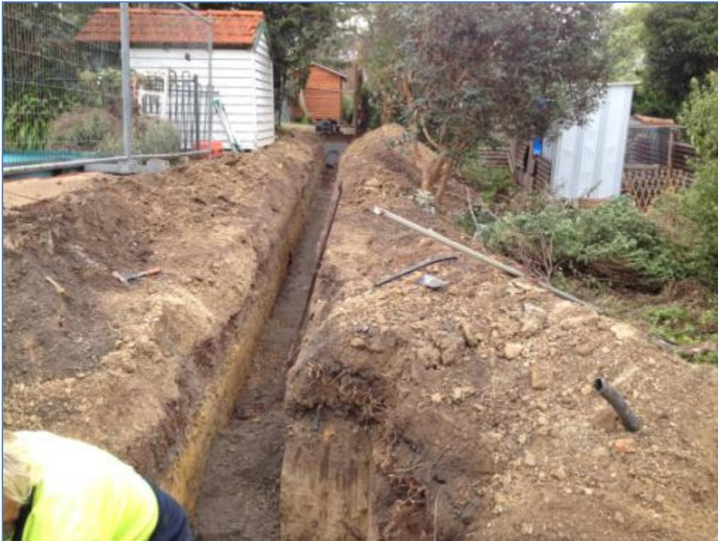
Figure 5 - typical easement drain trench along a side boundary
