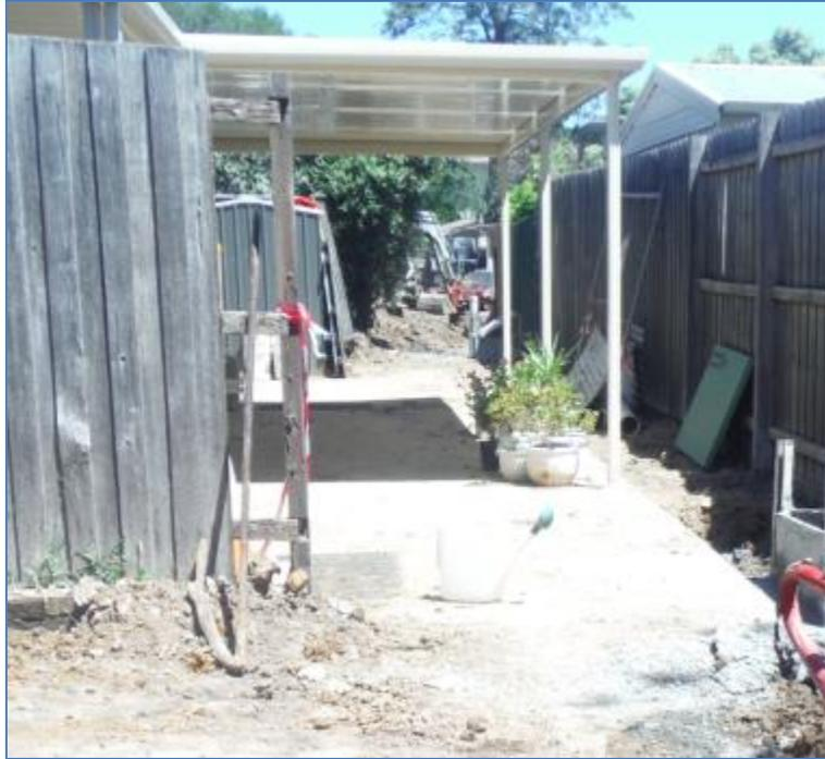
Figure 14 - a light weight, open and demountable verandah (typically approved). This location was subject to an easement drain renewal and the photo is during works.
