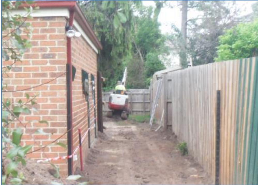
Figure 16 - excavator machinery often has a digging arm that raises, hence the need for height clearance under eaves
