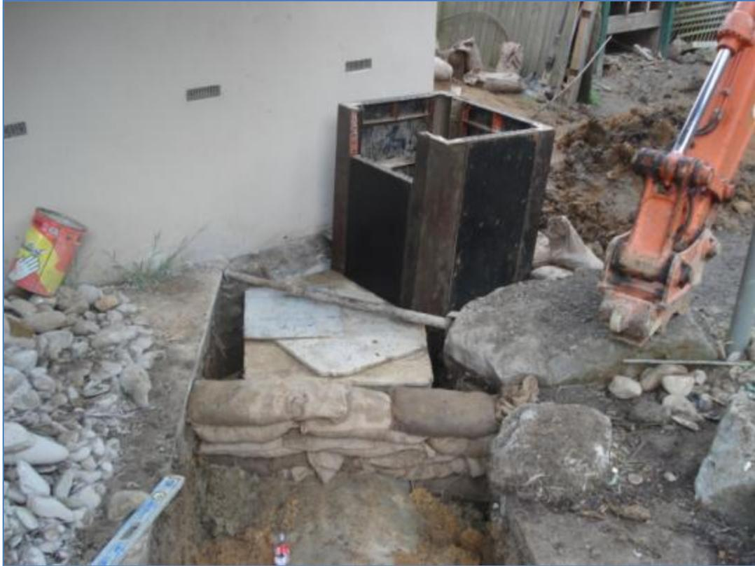
Figure 18 - major pit / pipe upgrade works in an established property (hard up against a building) in an easement
