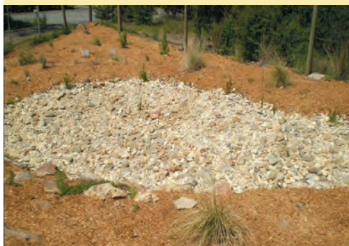
After: soil has been improved, dry-river bed collects water, any overflow will run into garden bed and be absorbed by wetland plants. The soil dug out of the dry-river bed pan was used to top up the lower bank.
