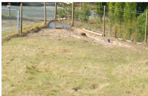
Before: poor drainage, water collects in the bottom corner, soil is compacted.
