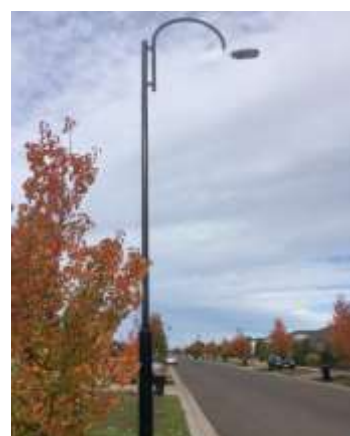
Figure 7: Example of a standard luminaire installed on a non-standard pole
