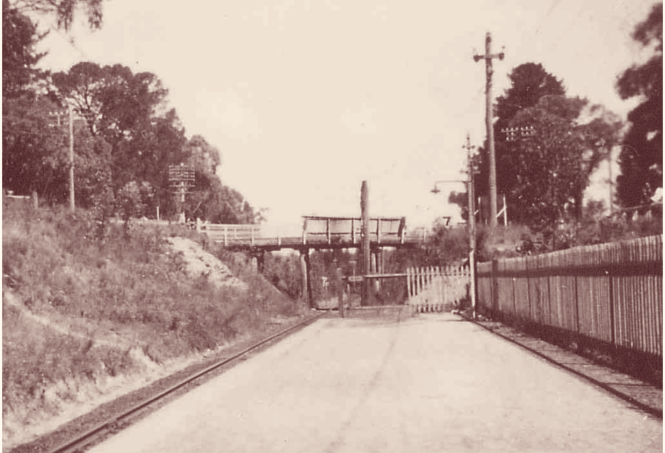
Heathmont railway bridge before it was replaced with a steel construction
