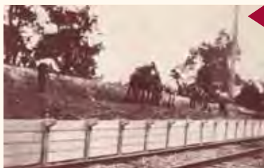
Building Heathmont railway station platform by Wieland brothers 1926, using horse and plough
