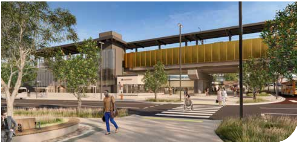
Looking towards the new Croydon Station from the pocket park on Main Street. Artist impression only, subject to change.
