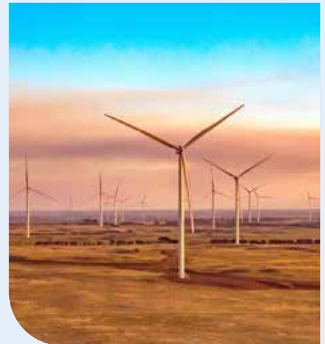
Renewable energy is being used to power Council-owned buildings and infrastructure.
