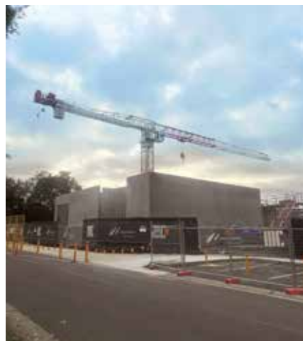
Works underway at the Croydon Community Wellbeing Precinct.
