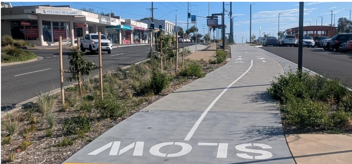
Figure 3 The new shared pathway along Railway Avenue, Ringwood East.
