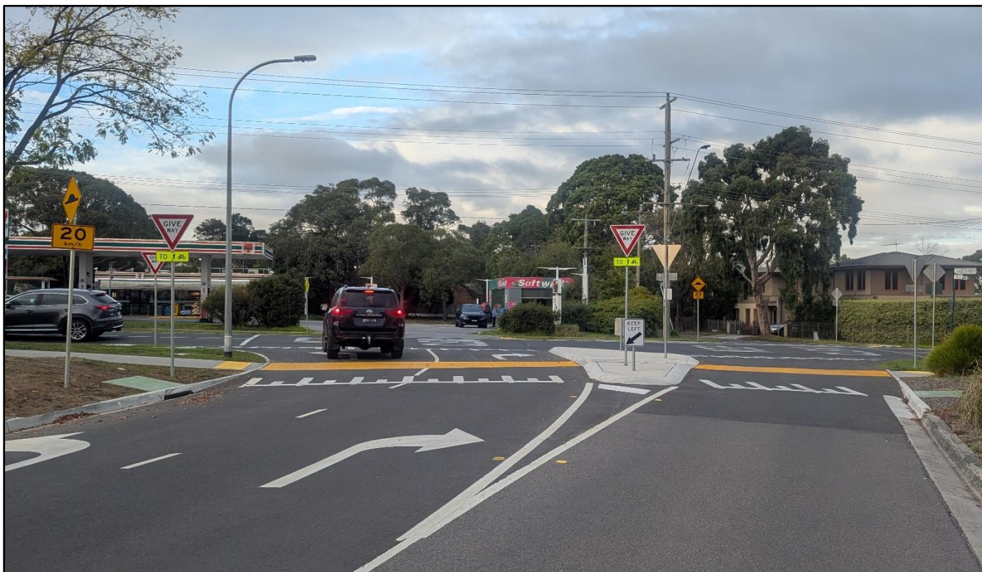
Figure 28 Shared path priority crossing, Golden Ridge Drive, Corydon Hills
