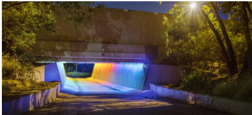
Lighting treatment, Larissa Underpass
