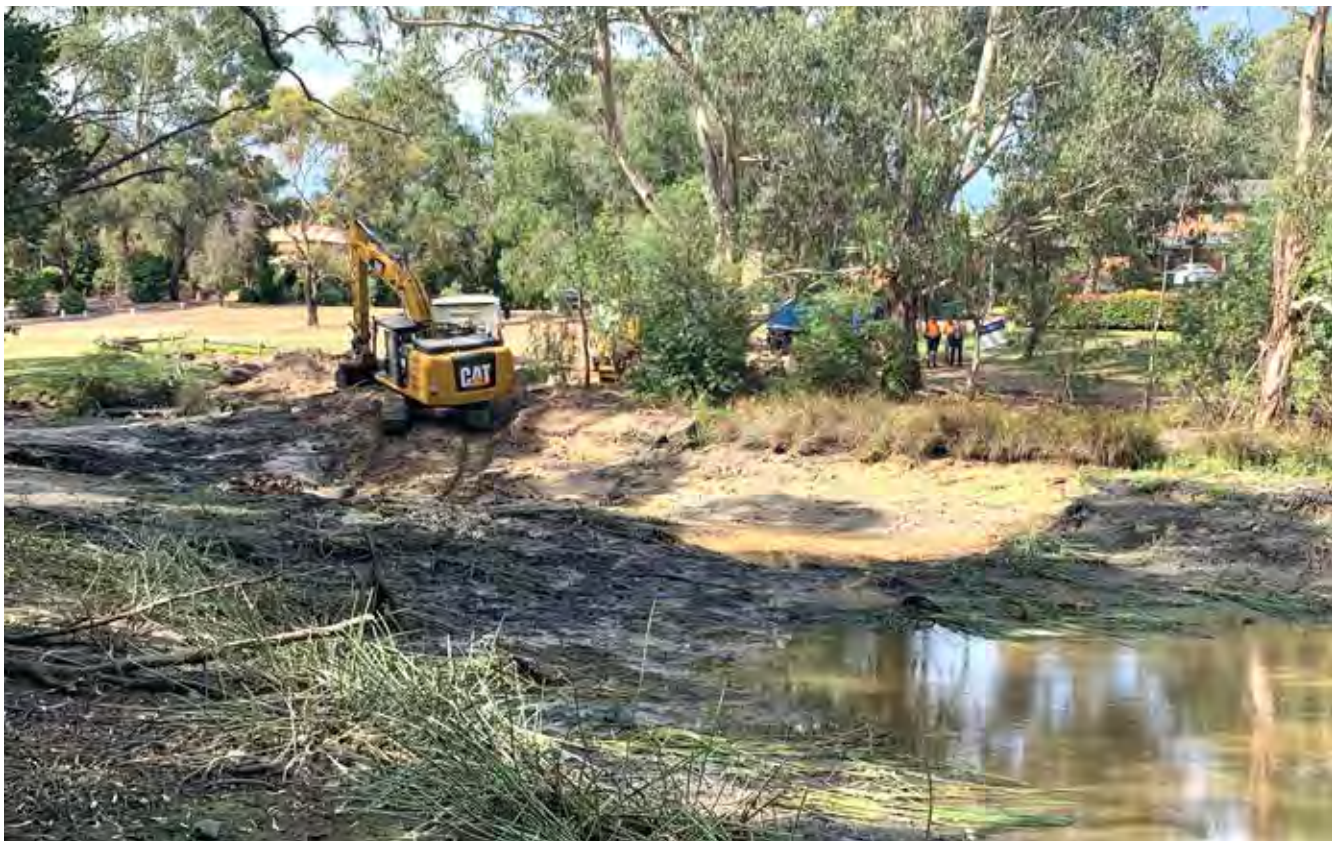
Desilting works at Settlers Orchard Reserve Pondage
