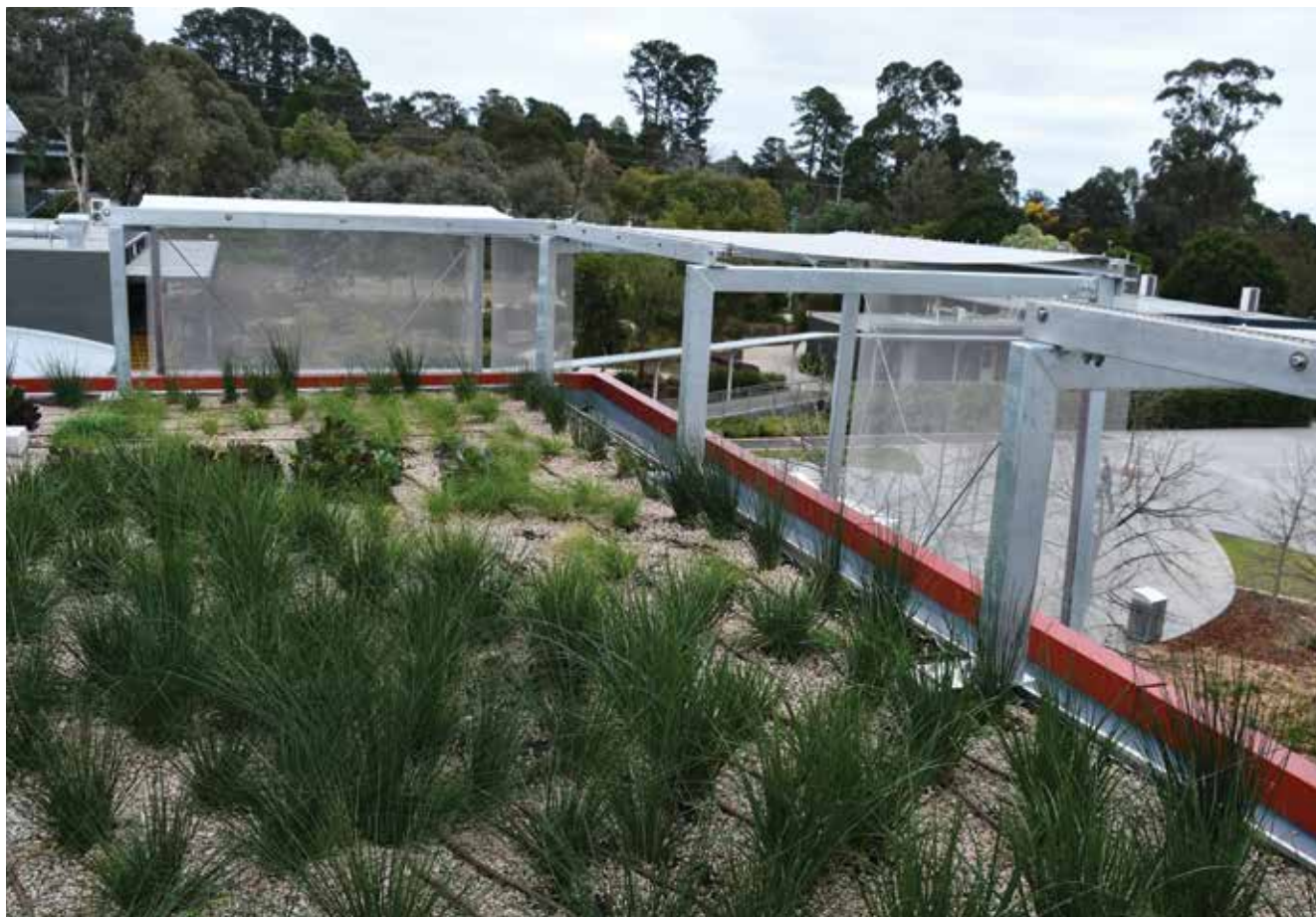
Yarra Valley Grammar in Ringwood has installed a rooftop garden on one of their buildings
