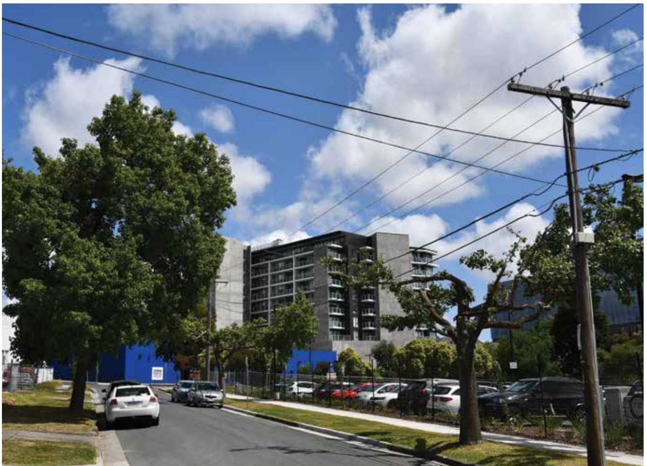
These trees in Pratt Street, Ringwood illustrate the competition for space between street trees and overhead power lines
