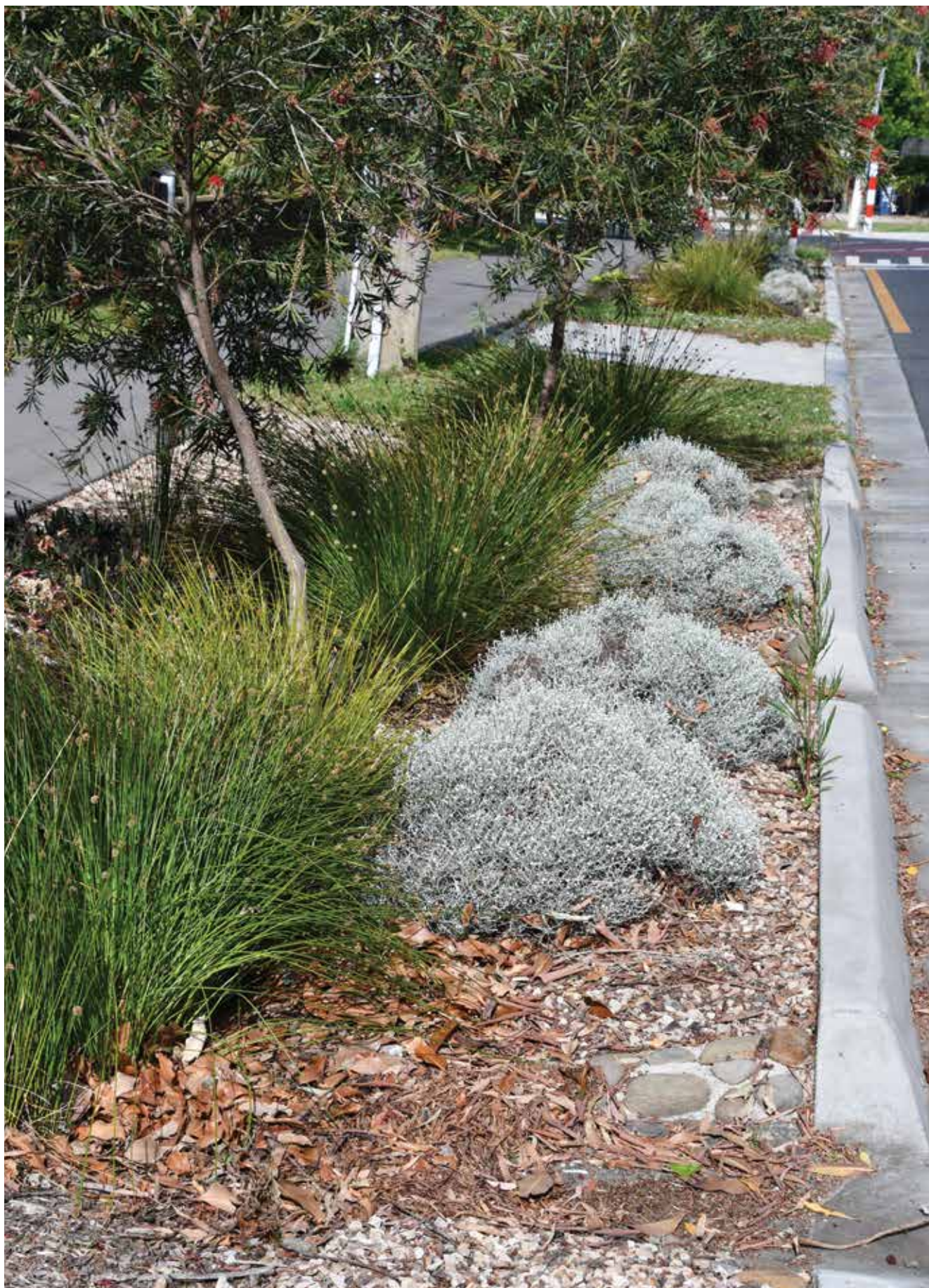
The water sensitive redesign of Knaith Road, Ringwood East enables stormwater runoff from the road to passively water vegetation in the nature strip
