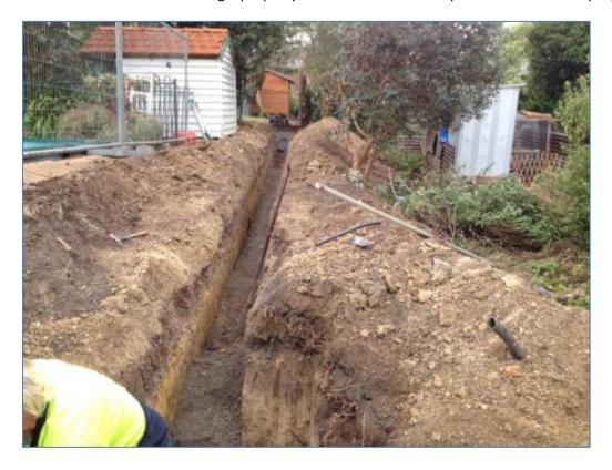
Figure 5 - typical easement drain trench along a side boundary
