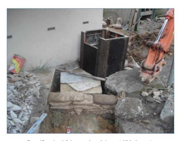
Figure 18 - major pit / pipe upgrade works in an established property (hard up against a building) in an easement
