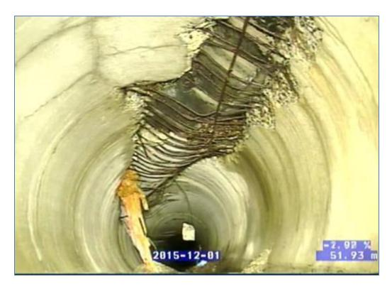
Figure 20 - an internal view of a drain that has failed and collapsed due to loading
