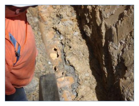
Figure 19 - a broken (old) terra cotta drain in an easement that needs replacing
