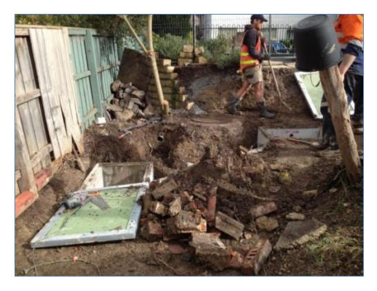
Figure 4 - Council contractors accessing a property to rebuild an old brick pit at the rear of the property
