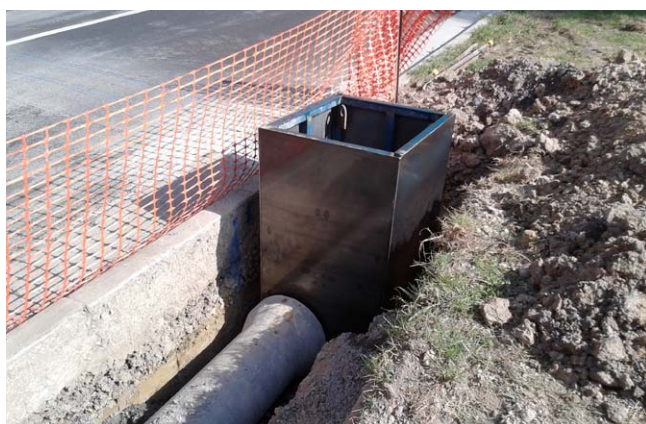
Figure 8 - New pipe and pit construction
