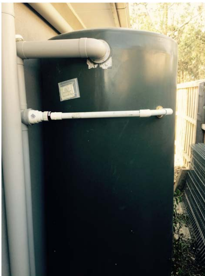
Figure 13 - Typical tank slow release orifice
