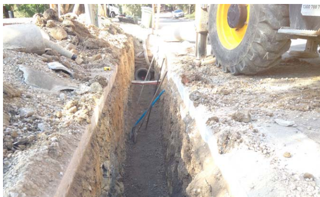
Figure 7 - Typical drainage trench pipe bedding
