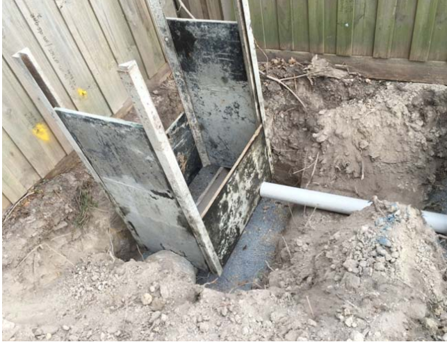
Figure 4 - Creation of a new pit over an existing drain
