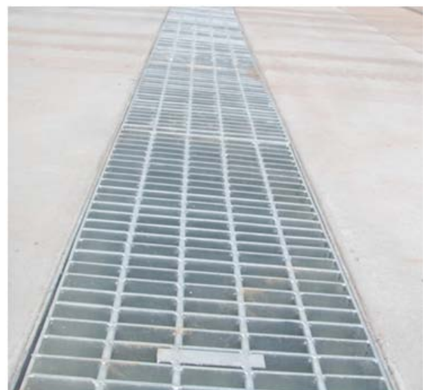
Figure 14 - Typical bike safe trench grate
