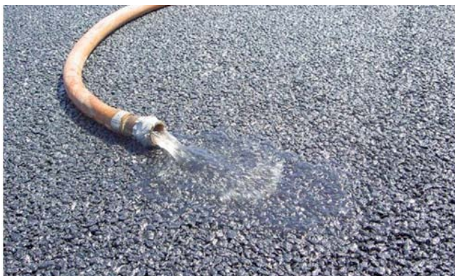
Figure 26 - An example of low impact pervious pavement
