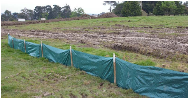
Figure 18 - Typical silt fence installation
