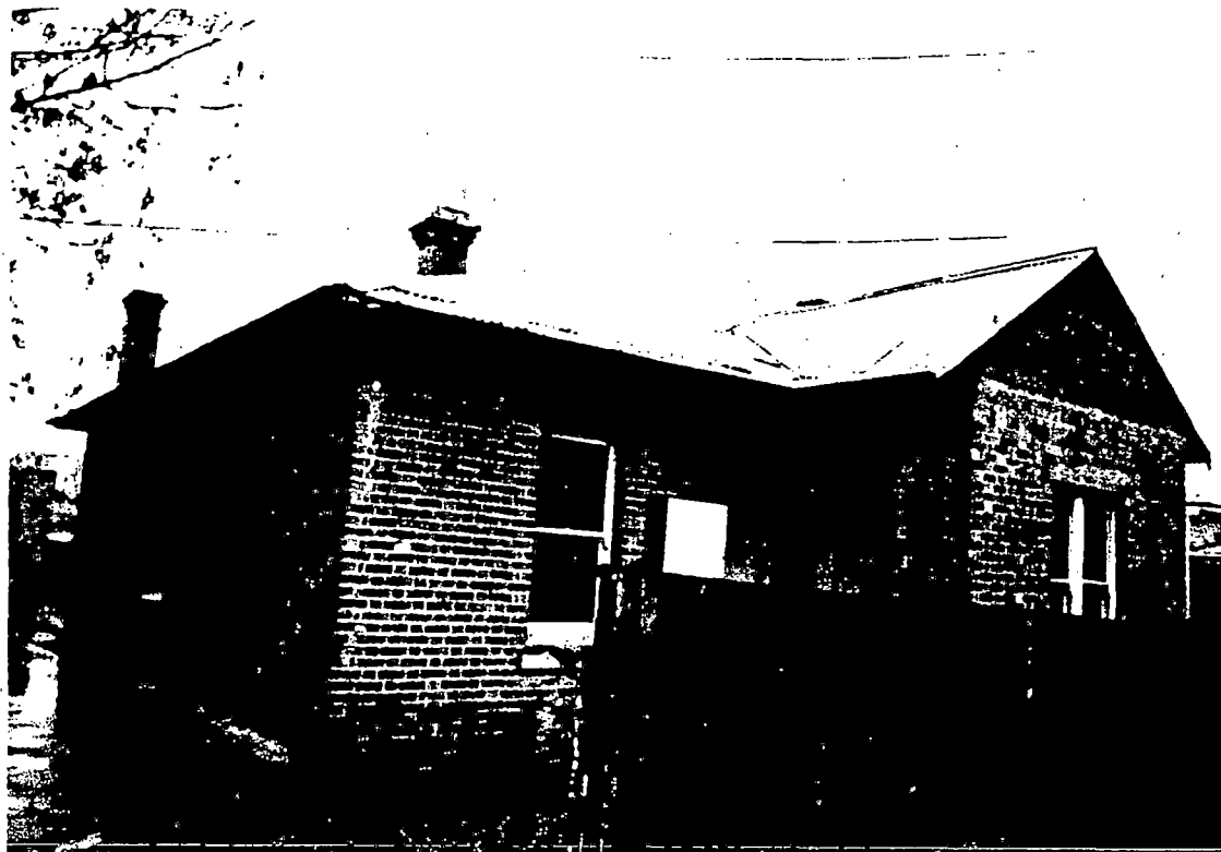
View from street (south east)
