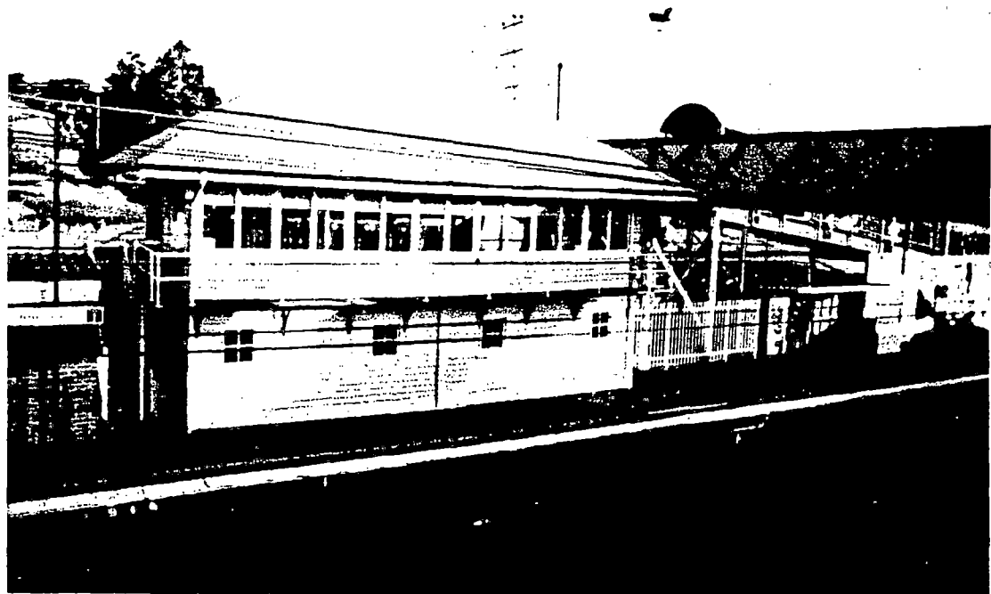
Signal box north elevation
