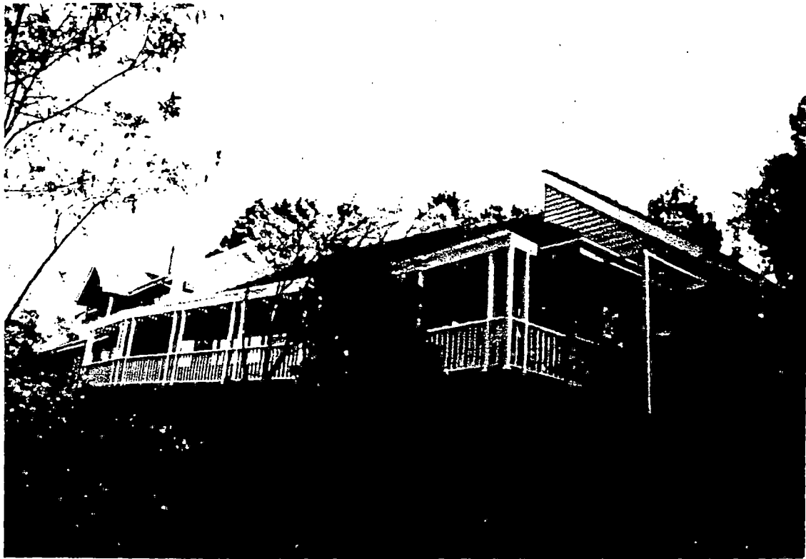
West elevation of addition from Alto Avenue
