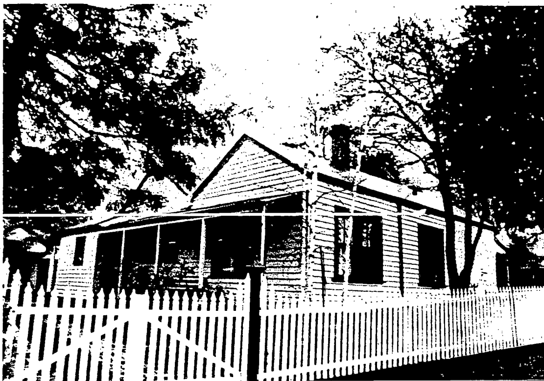
View from north east
