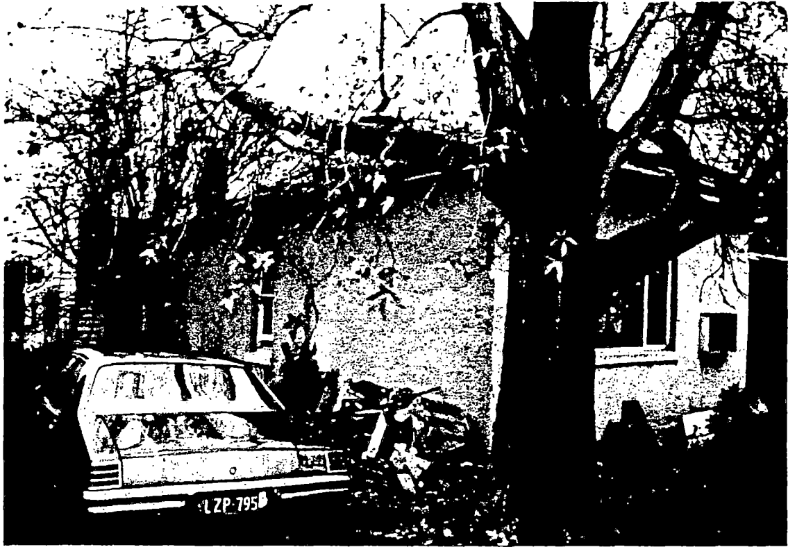
View from the street (south east)
