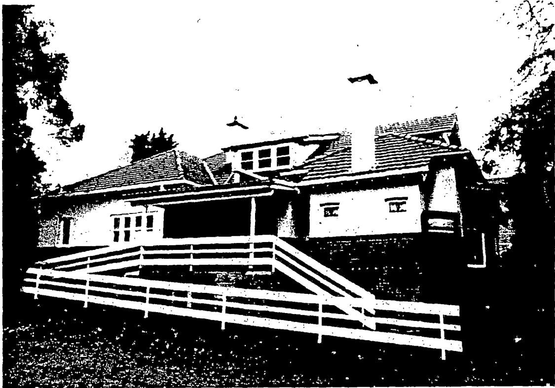
North elevation (facing carpark)
