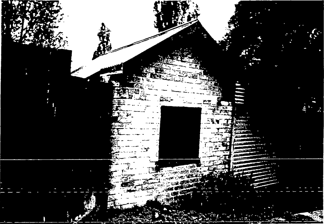
Brick shed from Barclay Avenue
