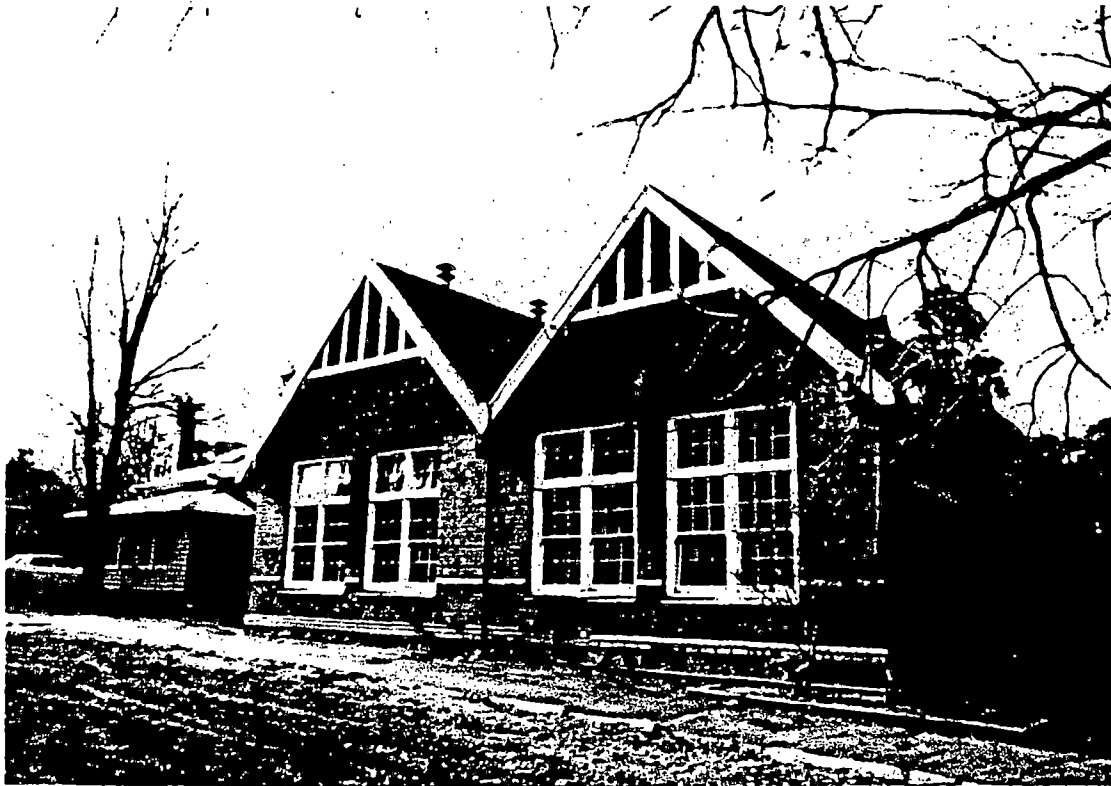
West Elevation from Anzac Street
