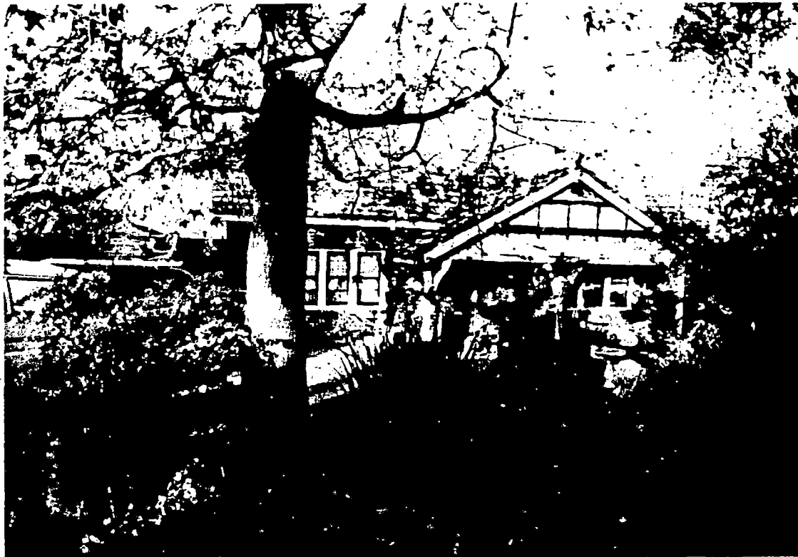
Street elevation from west
