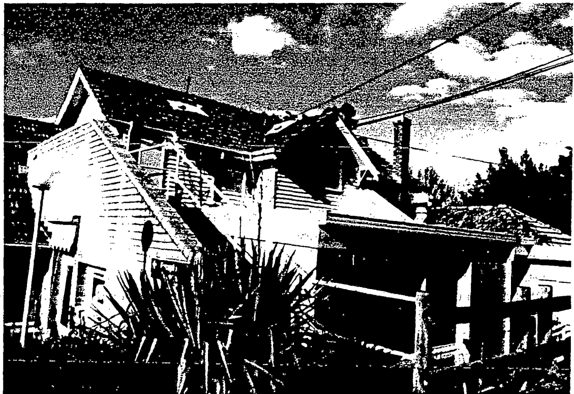
East elevation of addition from drive
