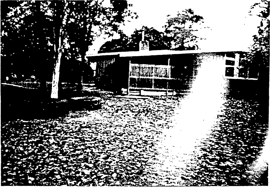
South west view
