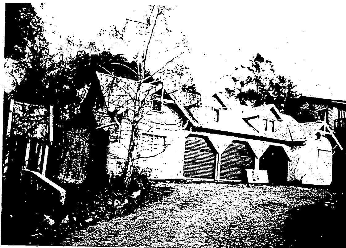
Former stables east elevation
