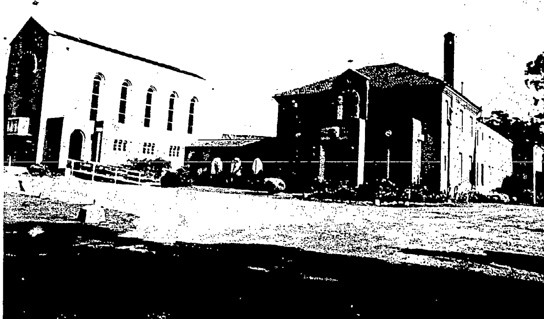
East elevation from north east
