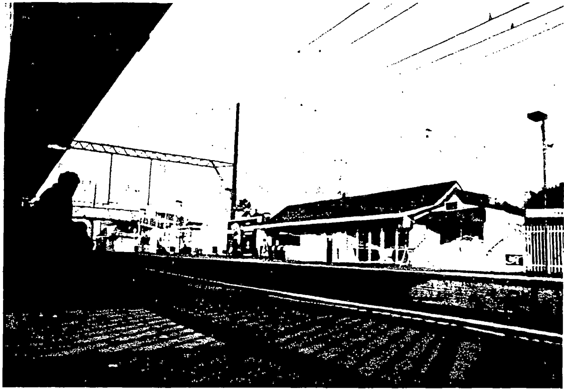
North elevation upside timber building
