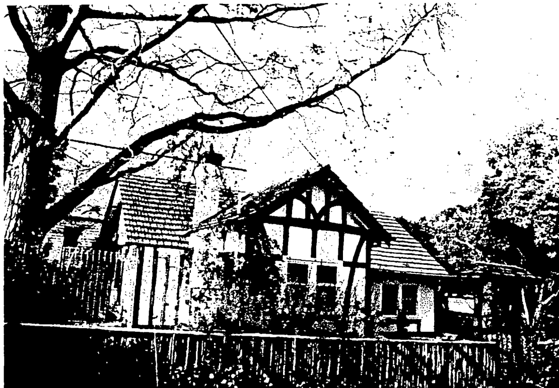
East elevation from Civic Square
