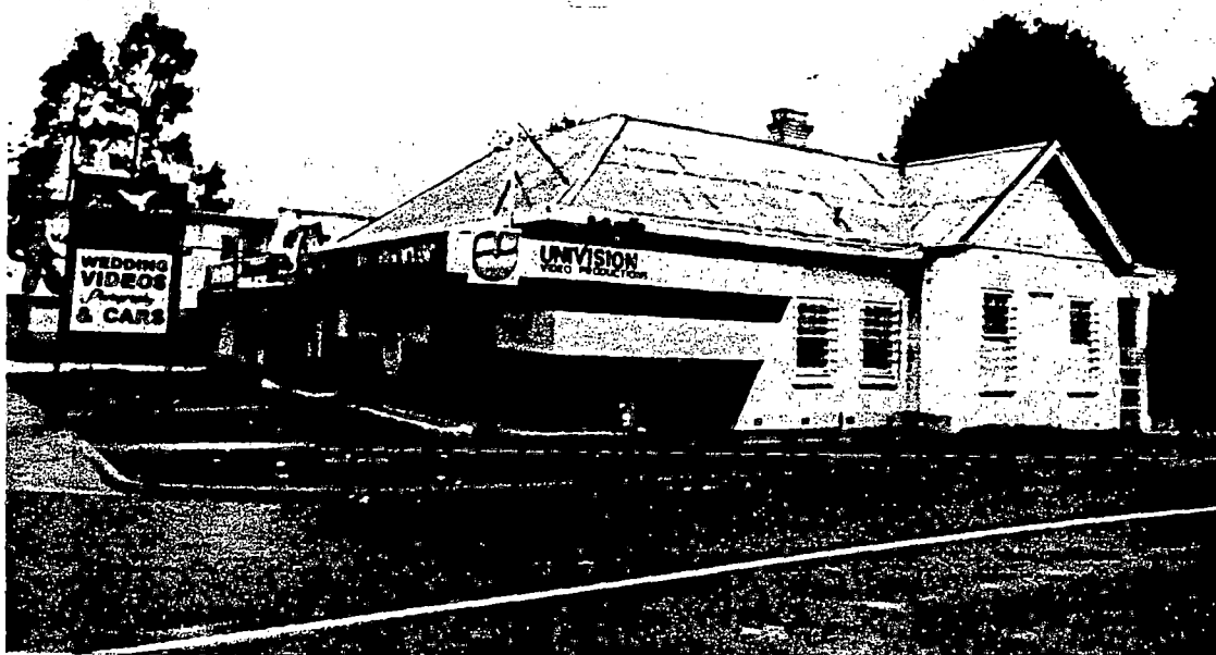
Street corner view
