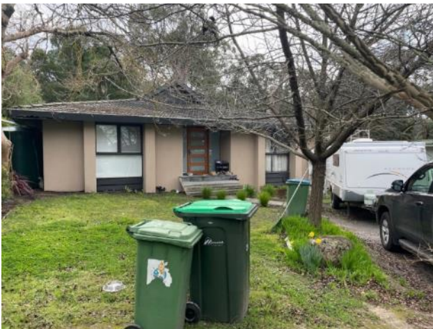
Figure 4 24 Rawson Court, Ringwood East
