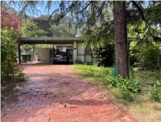
Figure 3 22 Rawson Court, Ringwood East
