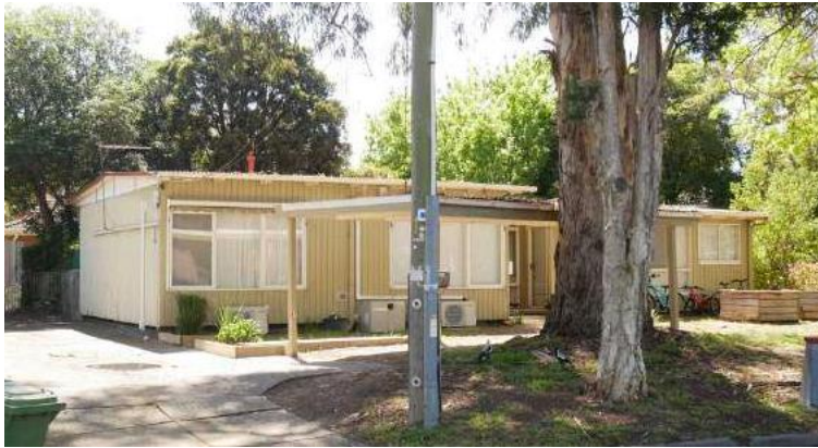
Figure 11 1/16 Valerie Court, Heathmont
