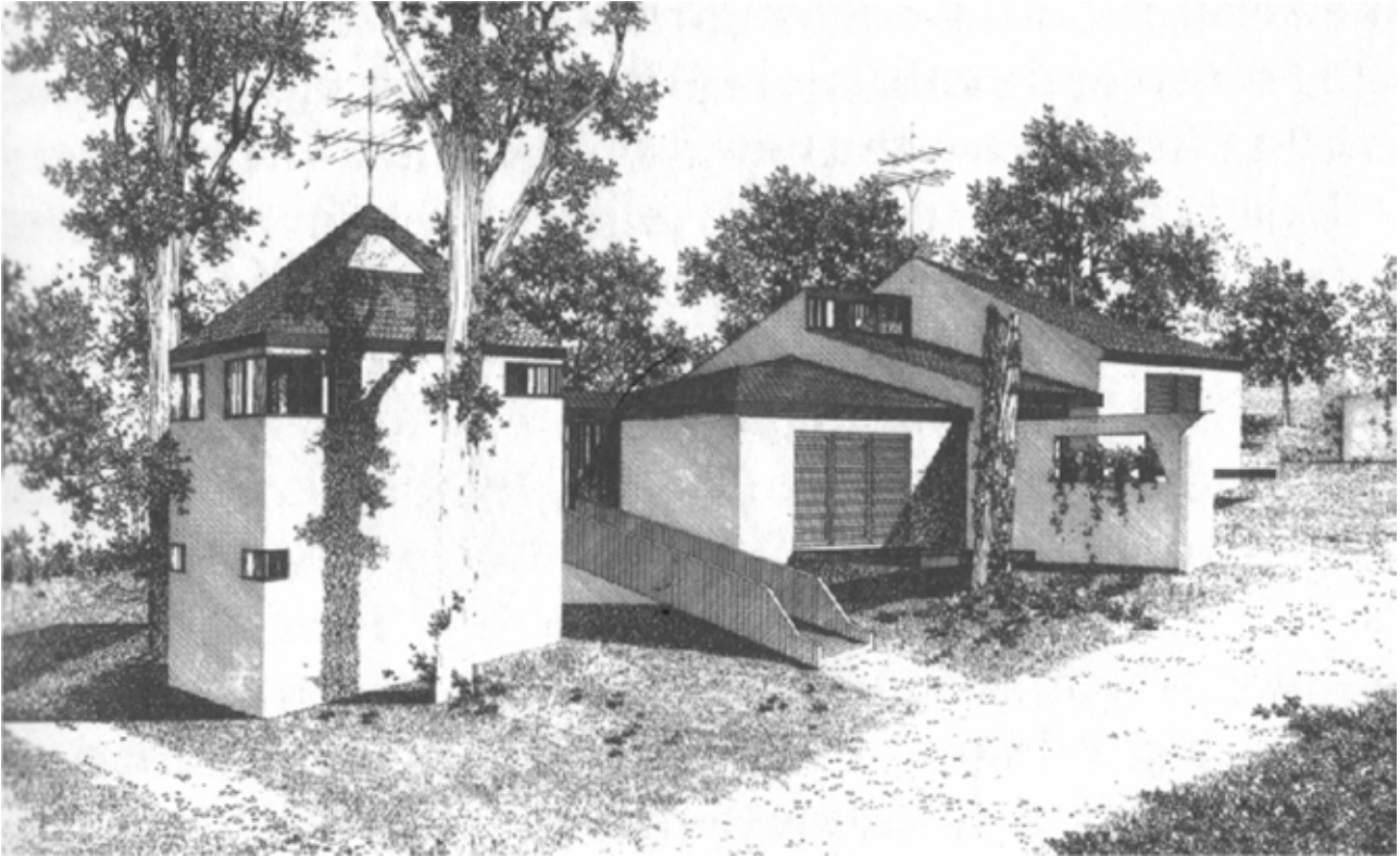
Figure 9e: The Kenyon House in Croydon (1964-74), the first house ever designed by Peter Corrigan (source: Conrad Hamann, Cities of Hope: Australian Architecture & Design by Edmond & Corrigan )
