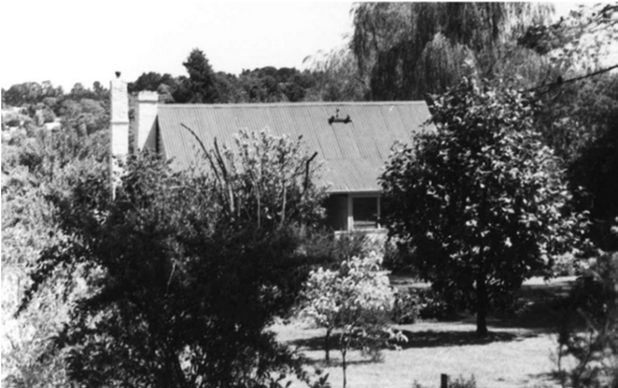
Figure 7d: Jenkin's Cottage in Croydon, recorded by the National Trust's photographer, John Collins, in 1984 (source: Picture Collection, State Library of Victoria)
