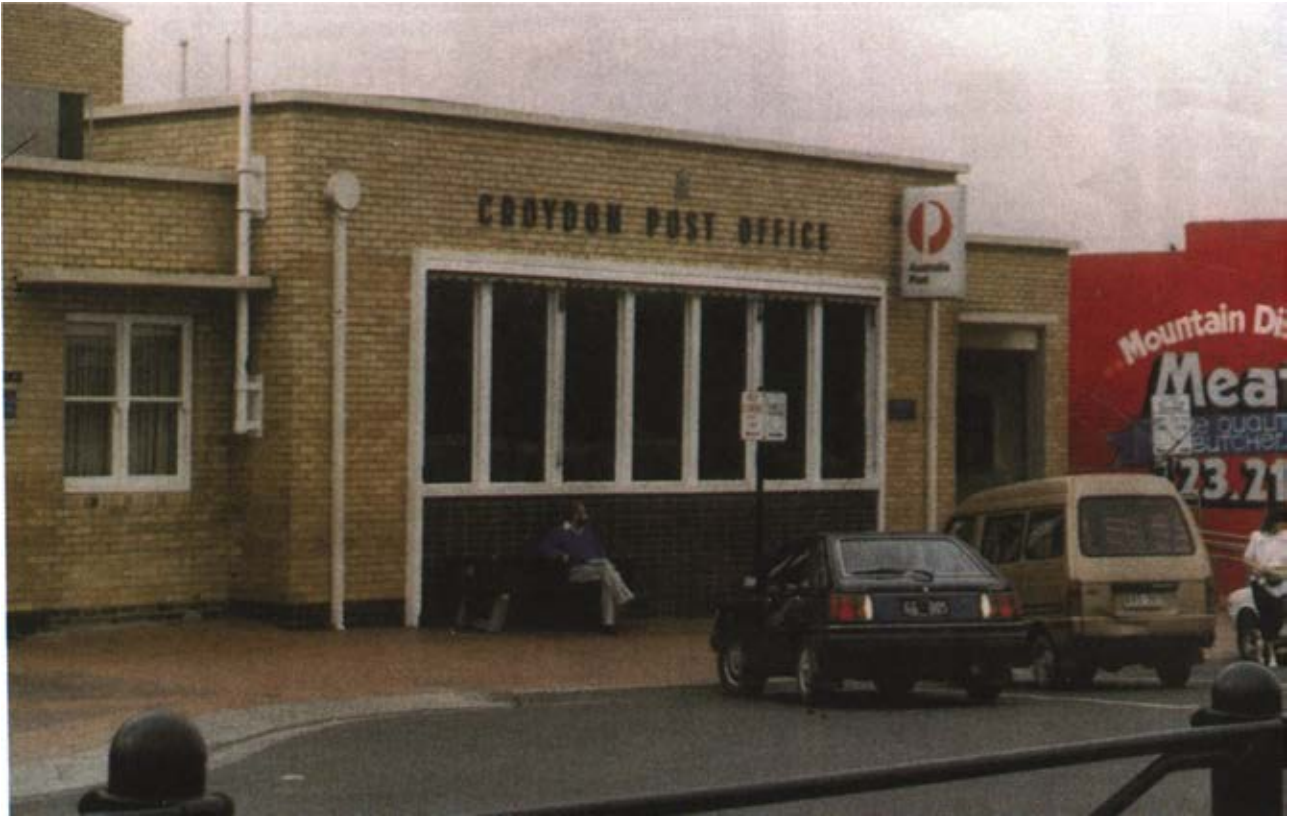
Figure 3c: Croydon's original purpose built-post office (1949), photographed in the 1980s (source: Croydon Historical Society, Croydon Then and Now )
