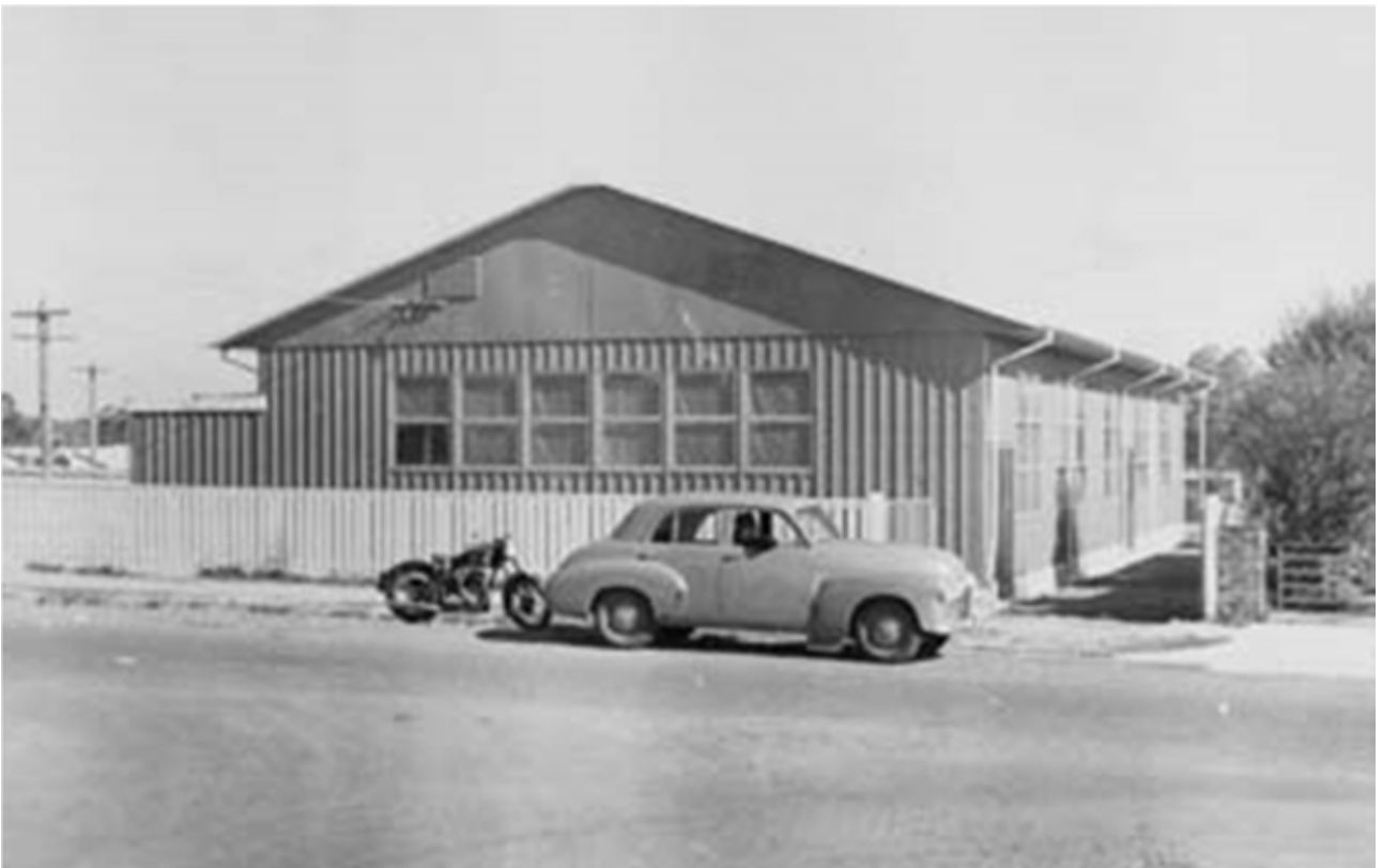
Figure 3d: The prefabricated aluminium building that accommodated Ringwood's telephone exchange, 1954 (source: National Archives of Australia)
