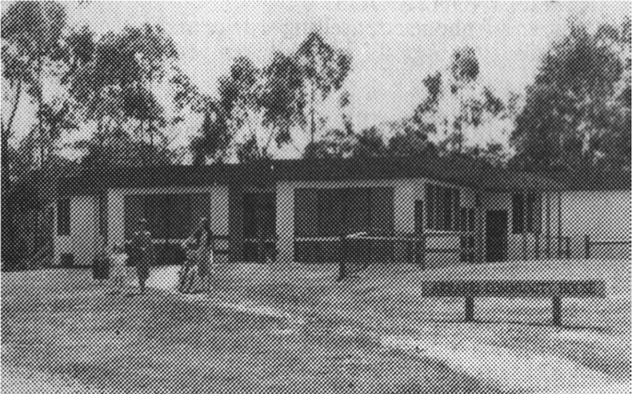
Figure 8i: The Arribri Community House in Bayswater North, soon after opening in 1983 (source: City of Croydon Community Handbook , 1984)
