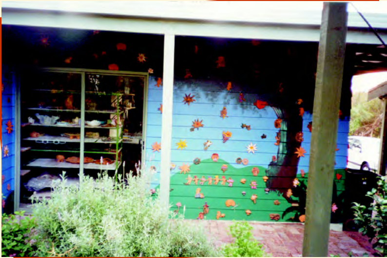
Exterior of Pottery “shed” prior to renovations
